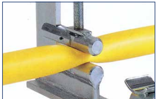
Picture 1.1.11 - The squeezing of PE gas pipe.
